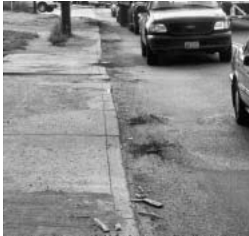
The existing asphalt surface on Broadway Street was severely deformed from traffic and distressed from age.
