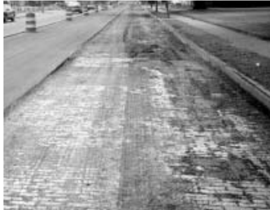
Severely distressed asphalt is milled to the bricks in the curb lane while the center lane is milled for a single course inlay.
