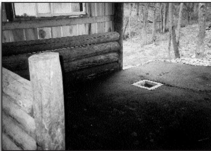
Andy Patterson's asphalt lined hog pen.
