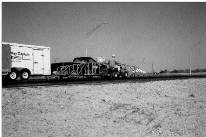
The Valley Asphalt Corp. takes profilograph readings that show the HMA pavement surface on the Butler Regional Highway is extraordinarily smooth.
