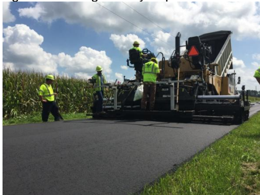
Figure 1: Paving Thinlay Asphalt.
